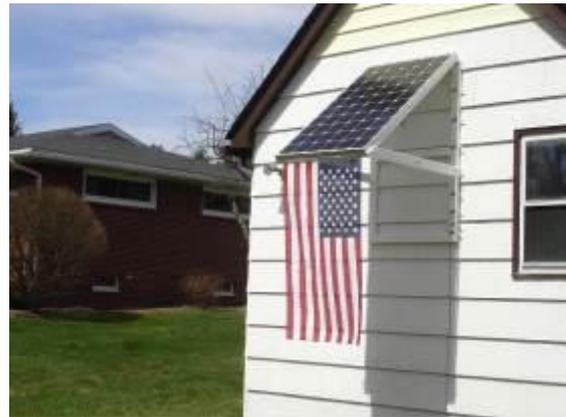
Figure 3: Module (255 W, 60-cell) mounted on back wall of house and inclined 40° from the horizontal (tilt appropriate for spring season).
